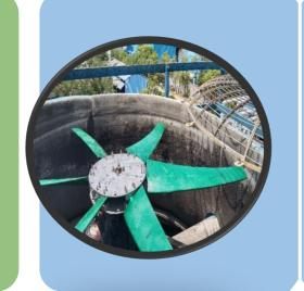
E Glass Epoxy FRP Blades for Cooling Towers
